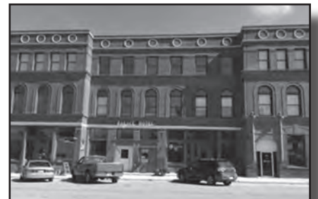
We were able to visit the historic Palace Hotel which is being renovated into apartments.
